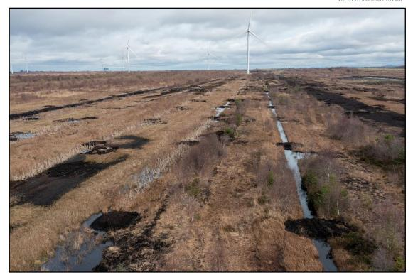
Photo 2-3: Peat dams installed on cutover bog within the Cloncreen windfarm site
